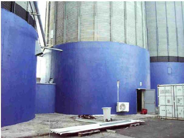
Figure 4. : Tank near the sea - Case F.
