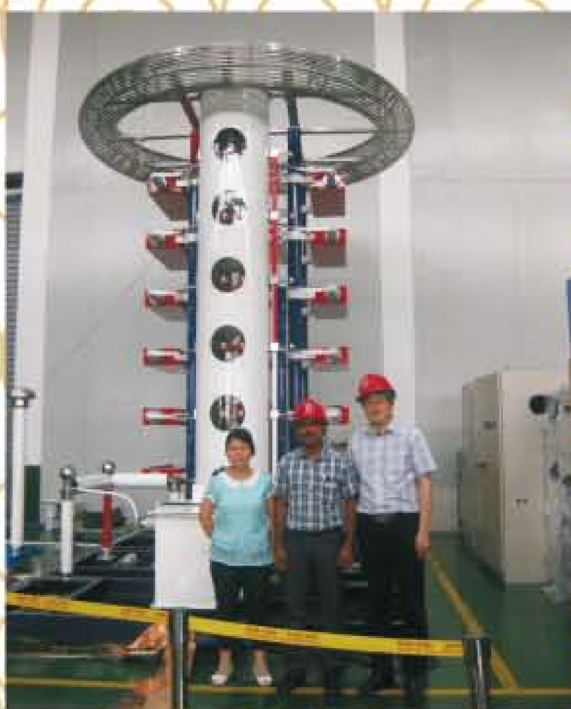
1200kV/60kJ for Cable Manufacturer
